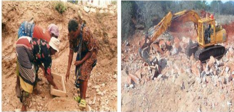
Fig. 6: women working in the mine without protective clothing and an excavator in a mining site
